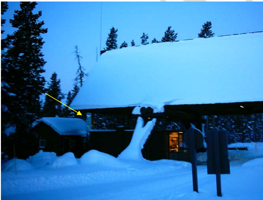
Figure 6. Ventilation duct to West Entrance kiosks
