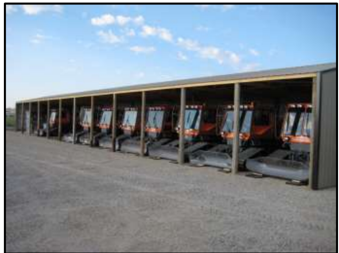
Photo 5: Groomer storage building example
