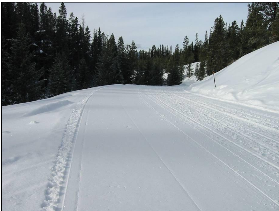
Photo 1.8 Trail grooming builds a solid, compacted base
